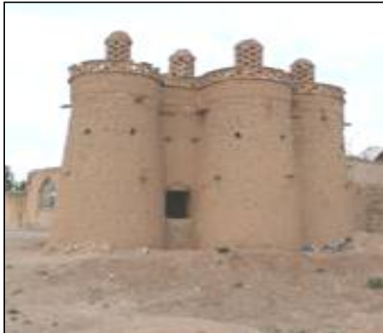
Fig. 7. Karkvand five-lobbed dovecot in Najafabad, dovecot, Mobarake(authors, 2013).
