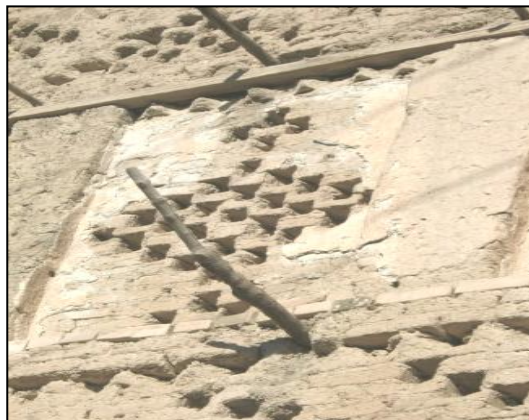
Fig. 5. The entering openings on the wall (authors, 2013).
