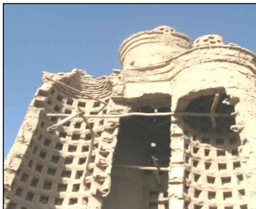
Fig. 8. The interior and the roof rim of a four-lobbed dovecot, Jochi Isfahan (authors, 2013).
