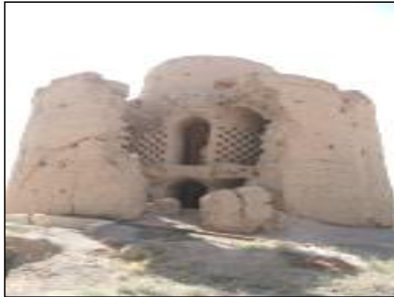
Fig. 1. A dovecot consisting of two concentric cylinders, Rahimabad (authors, 2013).
