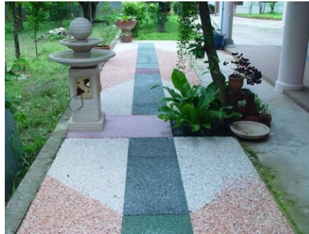
Fig. 7. Environmental friendly concrete block for cover of gutter surrounding the house.
