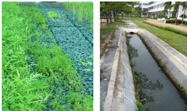
Fig. 8. Hydroponic cultivation and irrigation channel application with environmental friendly concrete block.
