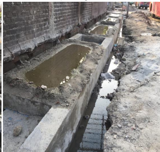
d) Curing of drains
