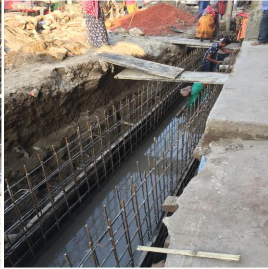
b) Casting of drain
