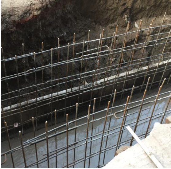
a) Reinforcement alignment of drain
