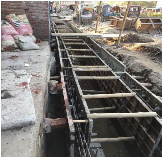
c) Frame work of drains
