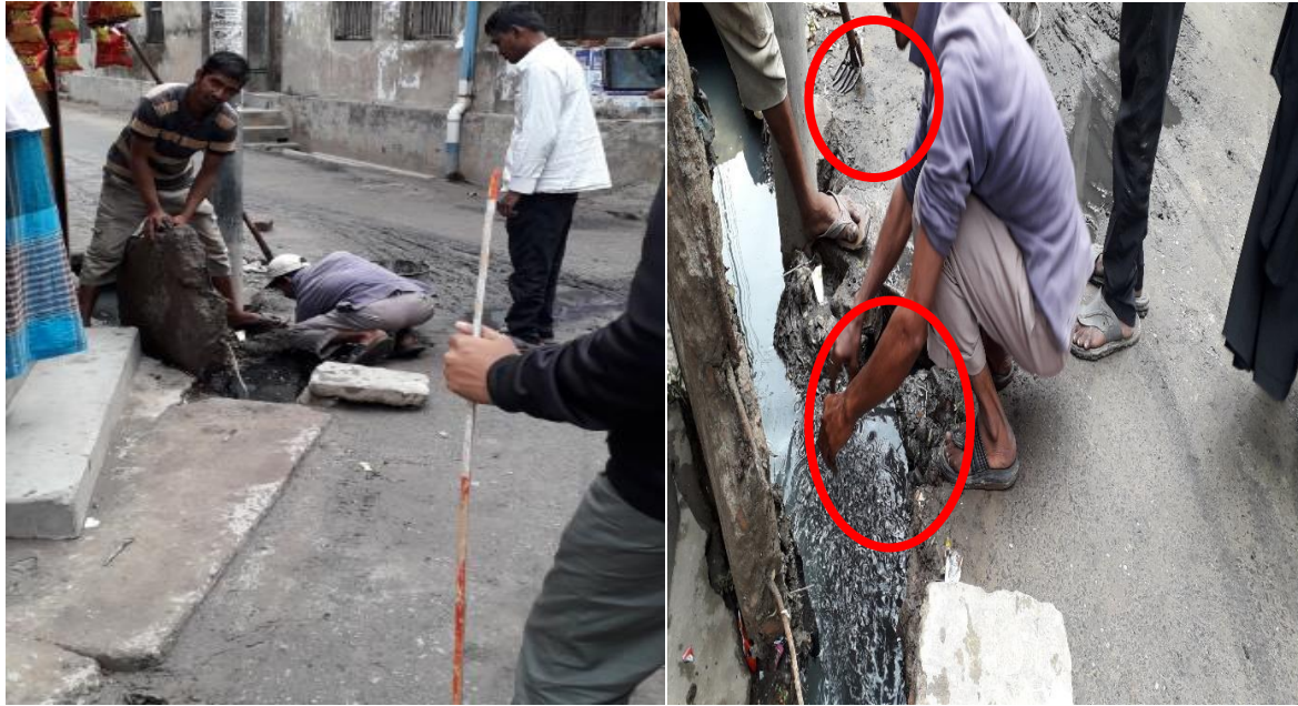
m) Cleaning of drains
