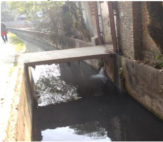
i) Slum on the bank of wide drain
