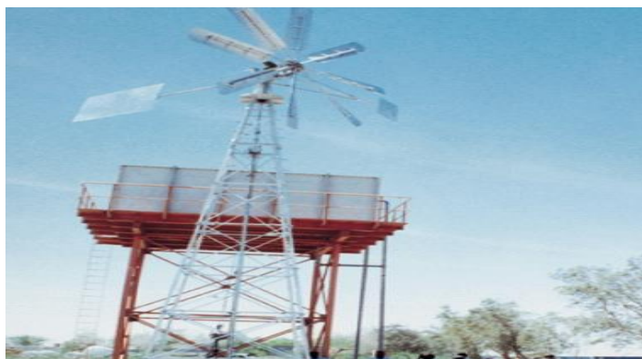
Fig. 8. Locally-manufactured wind pump installed at kilo 8 site.
