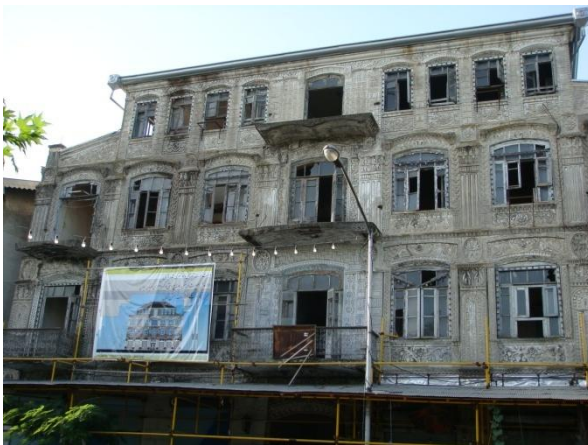
Fig. 8. the repair of historical building of Ministry of Justice in Anzali Port.
