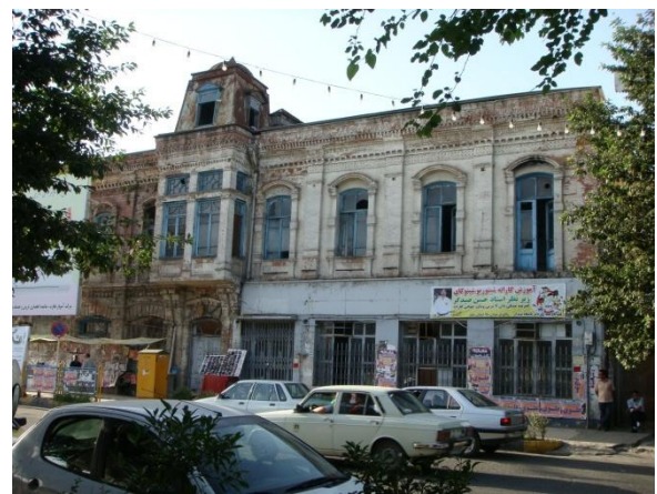
Fig. 9. a historical building in Anzali Port.
