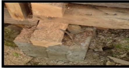
Fig. 6. Foundation – Jirnal, Gilan Cultural Heritage.
