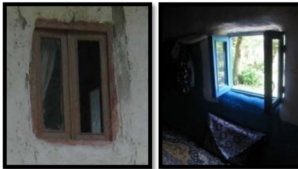
Fig. 22. Window Old.Detail, Gilan Cultural Heritage.
