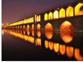
Allah Verdi Khan bridge
