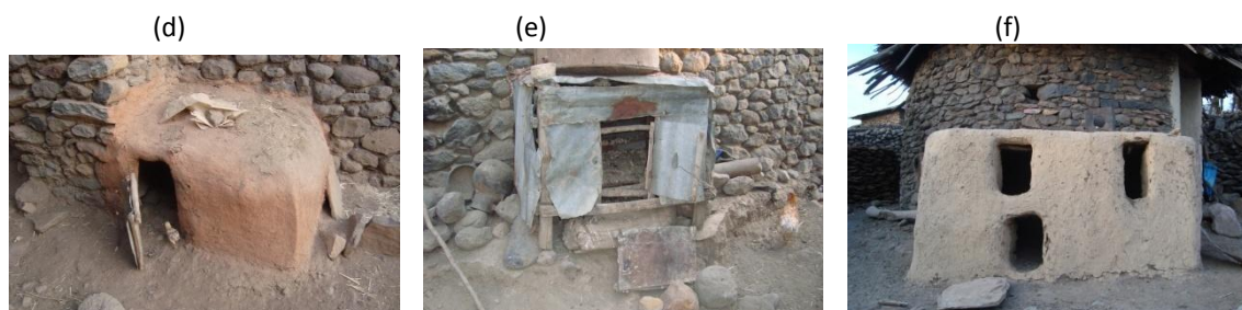
d= wooden cemented with mud, e= iron sheet type, f= mason type
